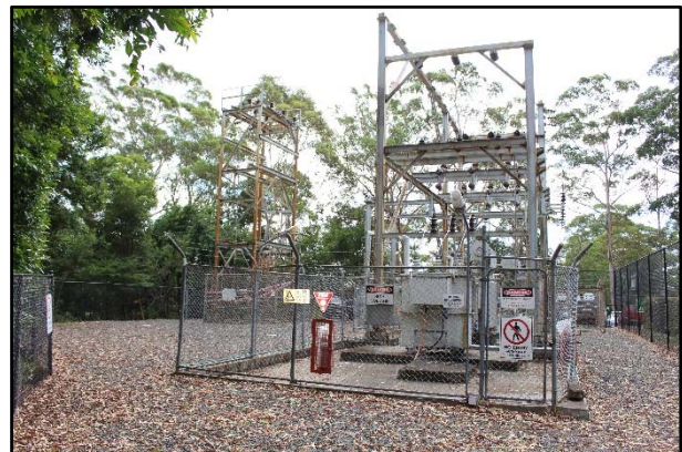
Plate 4: View of Substation from eastern entrance, west aspect. (Source: Niche 2018).
