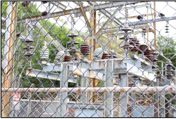
Plate 12: Example of modified grey ceramic insulators, south east aspect (Source: Niche 2018)
