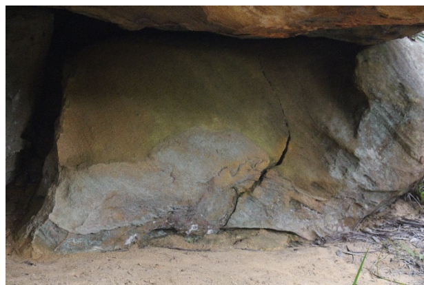
Plate 12: Subsidence related cracking to the northern side of the shelter.
