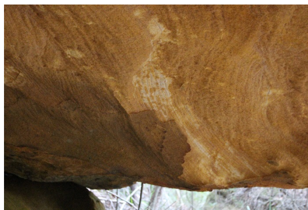
Plate 14: Subsidence related cracking to the northern side of the shelter.
