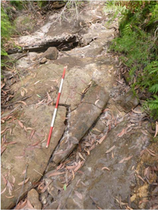
Photo 1: DA3B_LW11_008- Rock fracture, looking upstream along WC21. Taken on 14/01/2016.
