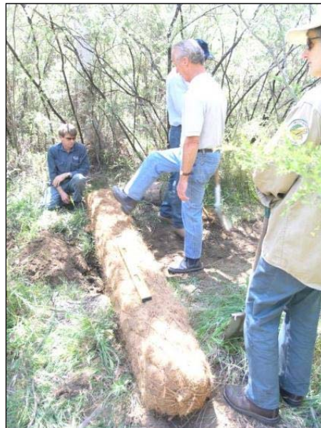
Figure 4-6 Round Coir Logs Installed to Spread Water
