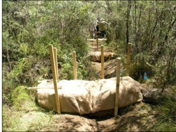
Figure 4-5 Small Coir Log Dams with Fibre Matting
