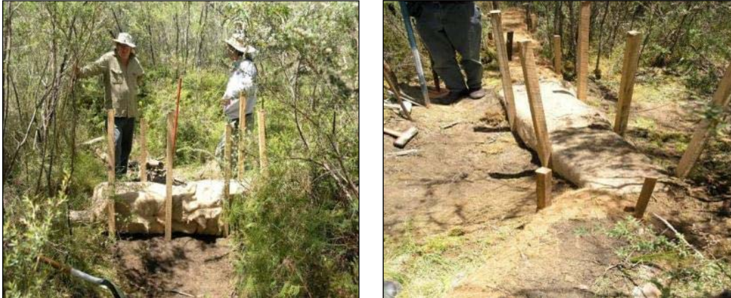
Figure 4-3 Installation of Square Coir Logs
