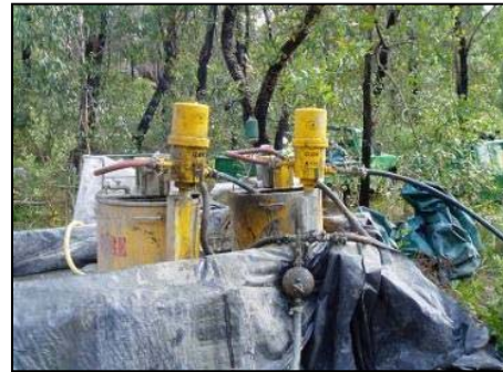
(b) Grout pump station setup
