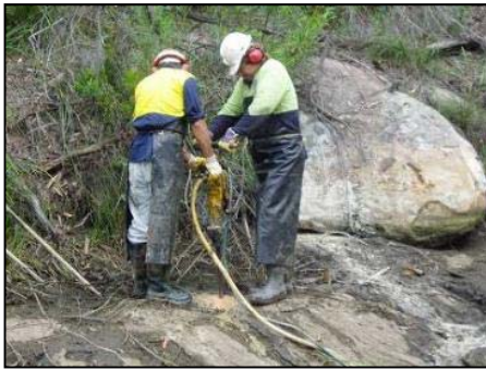
(a) Drilling into the bedrock
