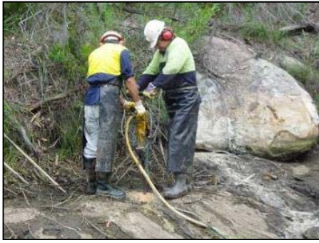
(a) Drilling into the bedrock
