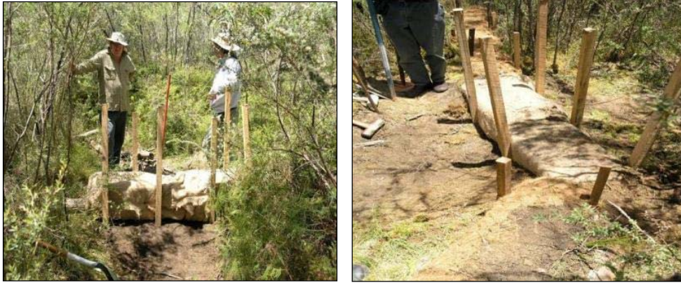
Figure 4-3 Installation of Square Coir Logs
