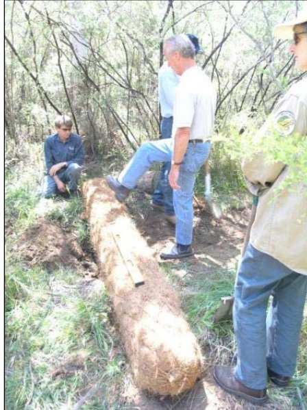
Figure 4-6 Round Coir Logs Installed to Spread Water
