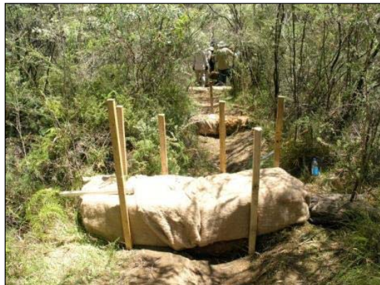
Figure 4-5 Small Coir Log Dams with Fibre Matting
