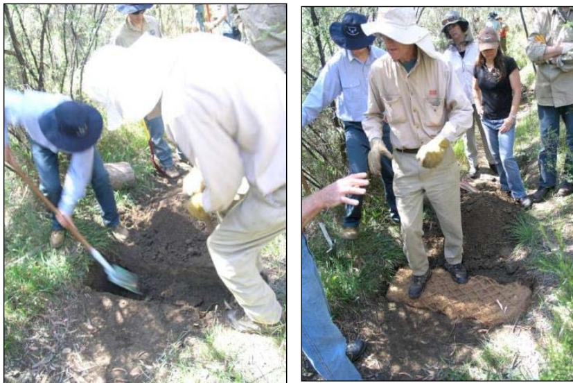
Figure 4-4 Trenching and Positioning of the First Layer of Coir Logs and Construction of a Small Dam in a Channel
