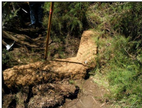
Figure 4-2 Square Coir Logs for Knick Point Control
