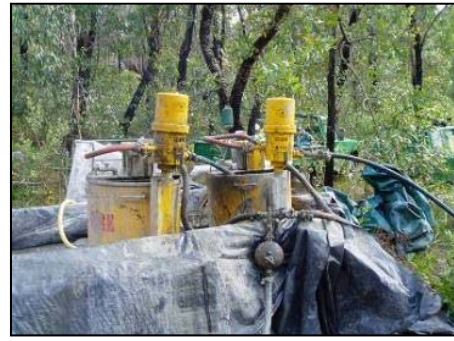
(b) Grout pump station setup
