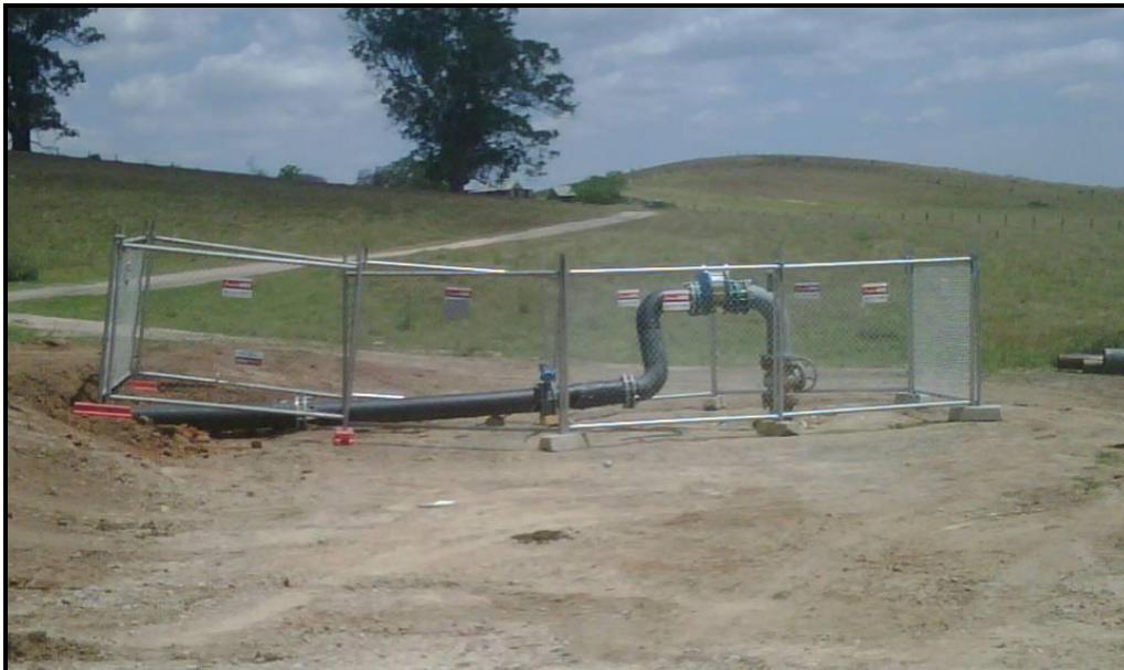
Figure 2.2 – Typical Wellhead
