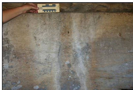
Plate 10: Another charcoal motif panel that has been impacted by water seepage
