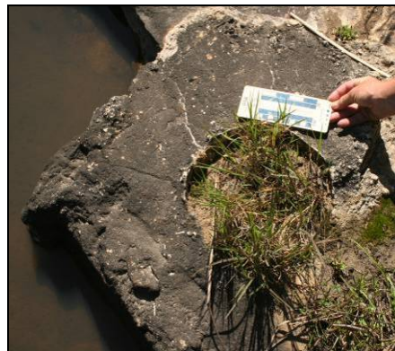
Plate 26: Former bridge post holes located in the sandstone, showing concrete packing, on the Georges River
