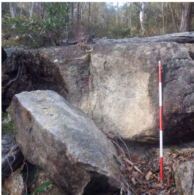
Photo 1: Overview of boulder fallen away from step. Taken 7/08/2023.
