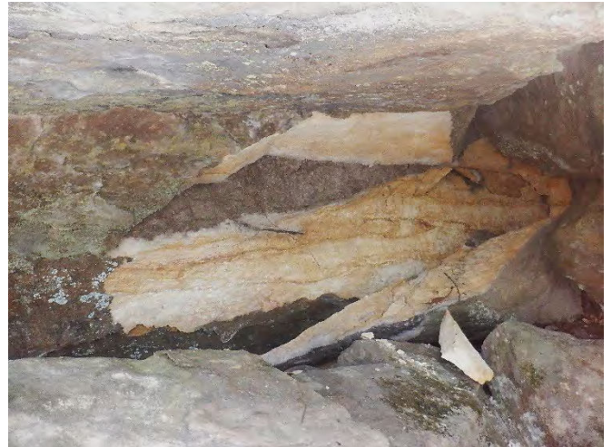
Photo 5: DA3C_LW21_026, close up section of rockfall. Taken 06/09/2023.
