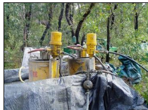
(b) Grout pump station setup
