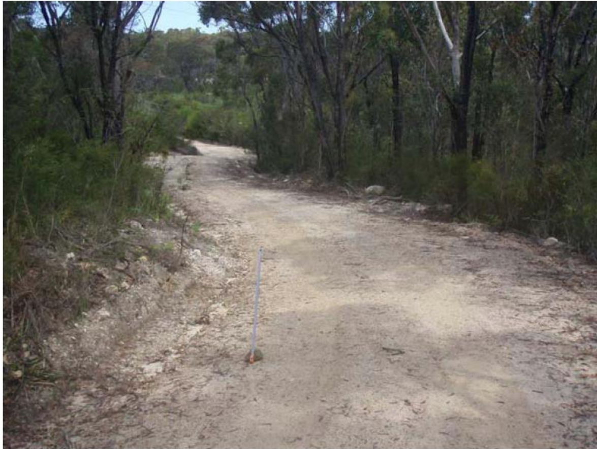
Fig. 6.4 Photograph of a Typical Fire Trail (Courtesy of IC)
