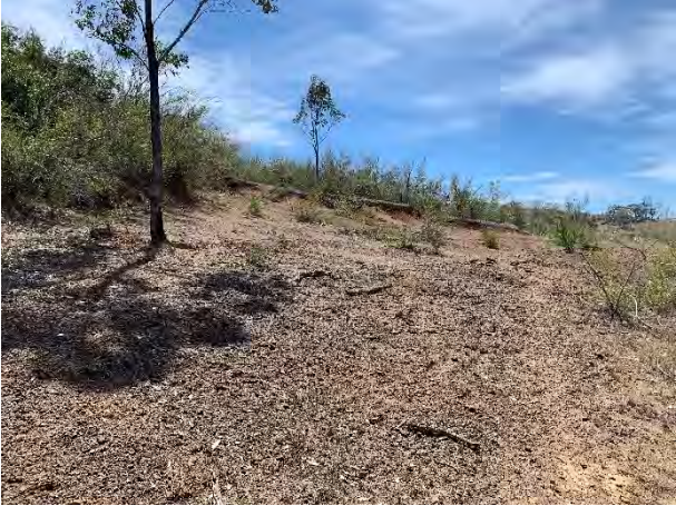
Area of erosion from photo point 7 during 2012, 2013, 2014, 2015, 2017, 2018 and 2019.
