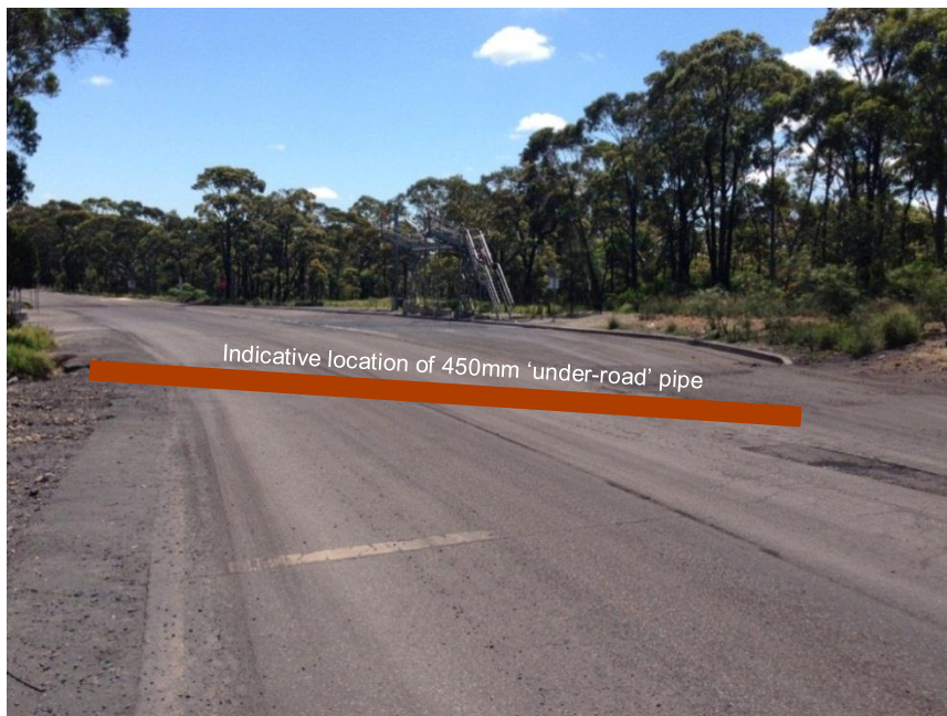
Figure 16: Indicative Location – sub-surface drainage pipe
