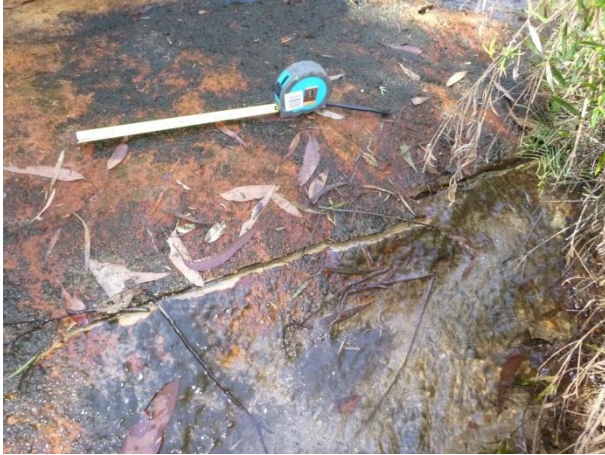
Photo 6: Impact DA3B_LW10_007 – rock fracture with reappearance of localised flow diversion. Taken on 18/11/2014
