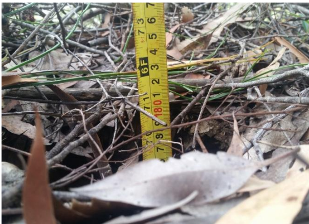
Photo 14: Impact DA3B_LW10_024. Depth of crack. Taken on 18/02/2015
