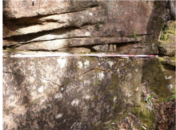
Photo 23: Impact DA3B_LW10_004 – Horizontal fracture on rock face. Taken on 27/10/2014
