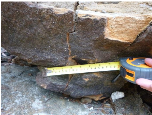
Photo 12: Impact DA3B_LW9_014 – Widest point of vertical fracture. Taken on 04/05/2015
