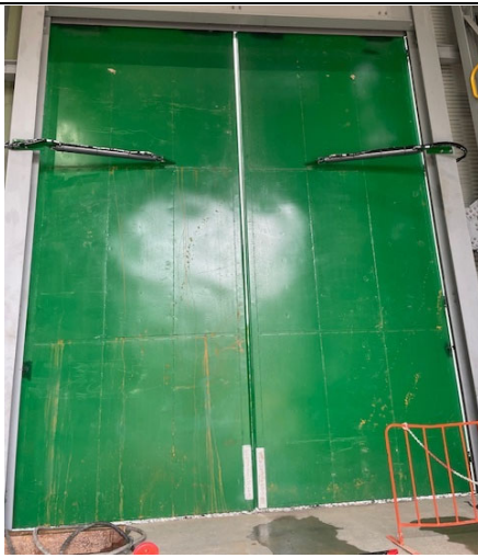
Plate 3: Heavy duty headframe doors
