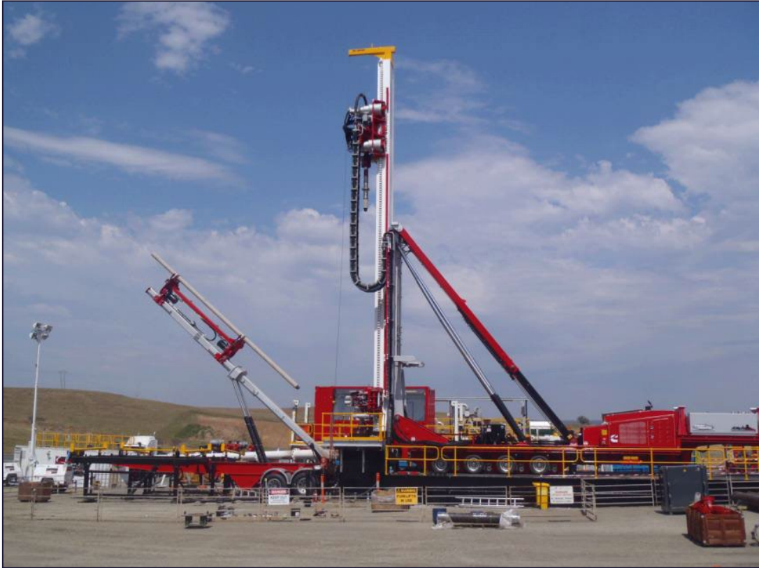
Plate 3: MRD Borehole Drilling
