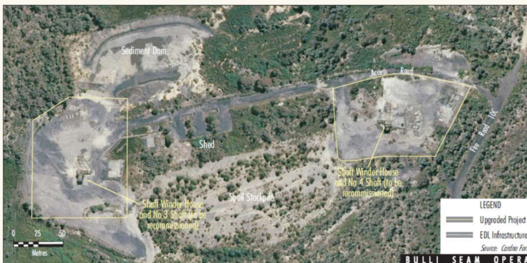
North Cliff Shafts
