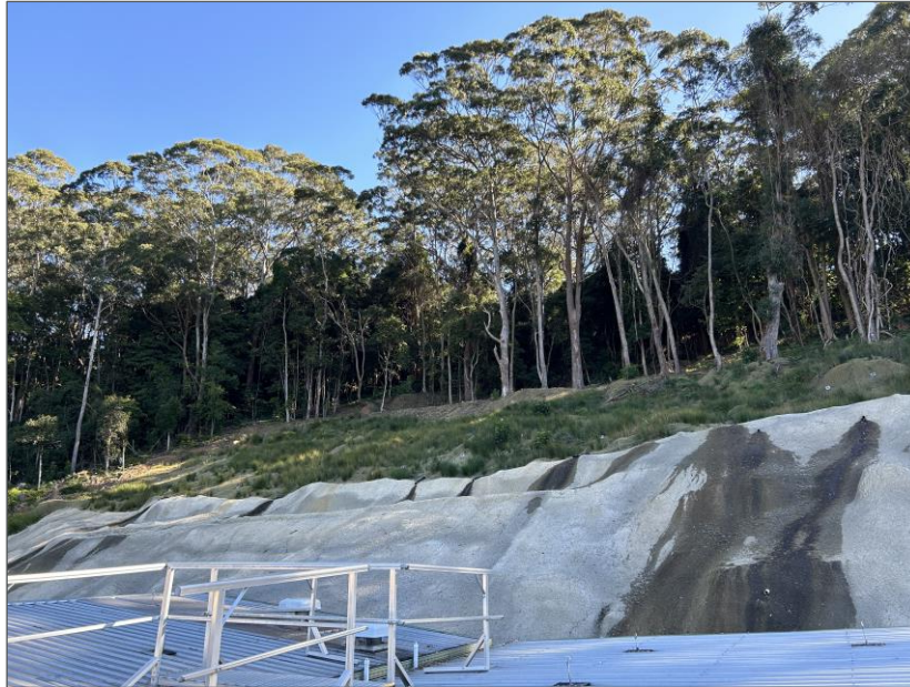
Plate 1 – Rectification Works Undertaken in Accordance with Special Condition E2 of EPL3241
